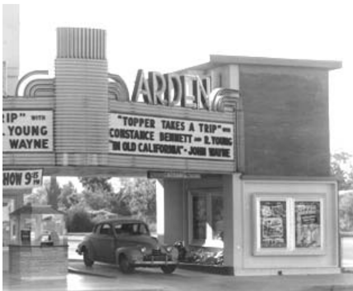
Arden Theatre, Lynwood California S. Charles Lee, Architect - 1942-47 Thin stone veneer on ticket booth and facade, planter box under poster cases in port cochere
