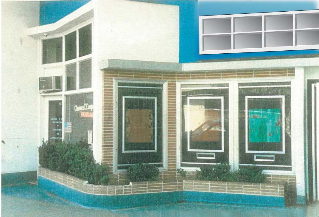
Reconstructed transom windows over entry doors
