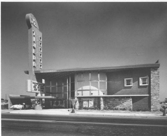
La Tijera Theatre, Los Angeles, California 1948-49 S. Charles Lee, Architect Thin stone veneer and planter boxes; asymmetric facade with drive-through ticket booth; title pylon and double sided signboard
