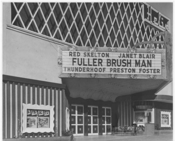
Helix Theatre, La Mesa, California 1947-48 S. Charles Lee, Architect Thin stone veneer planter boxes under poster cases; asymmetric ally placed ticket booth
