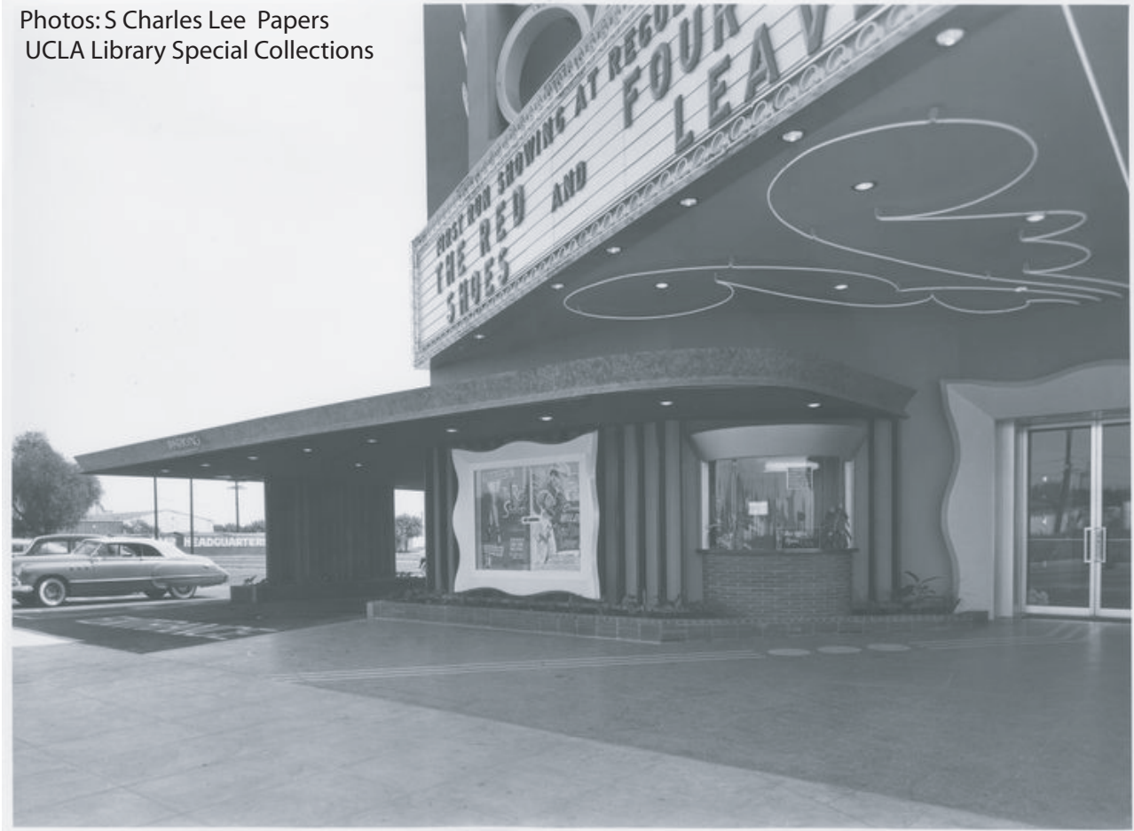
Garmar Theatre, Montebello, California S. Charles Lee, Architect 1949-50 (demolished) Brickvener ticket booth & planter boxes; asymmetric design with port cochure; patterned terrazzo
