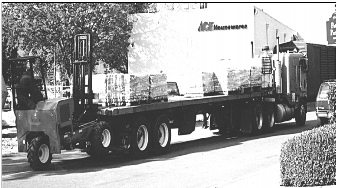
13.11. The third load of salvaged brick, Day 54 (November 10).
