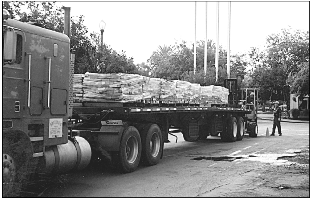
13.10. The second load of salvaged brick, Day 28 (October 2).
