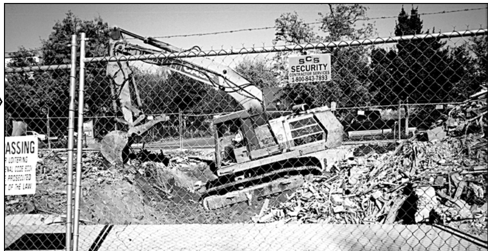
13.21. Bowers digging out basement concrete.
