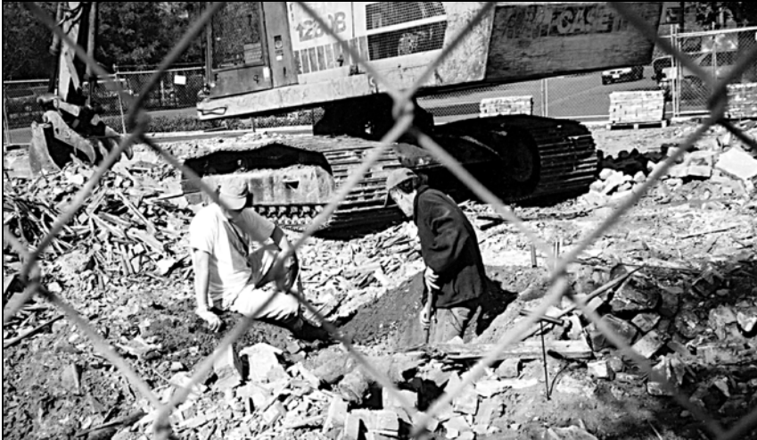
13.27. Two men digging for artifacts on the site, Day 49, Sunday, November 5.
