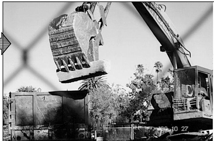
13.25. Loading a truck-sized piece of foundation/basement concrete.
