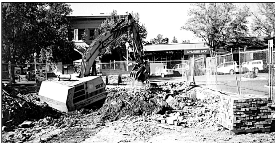
13.22. Pulling out the concrete foundation of the G Street wall.
