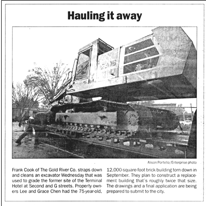
13.36. Davis Enterprise coverage of the excavator's departure, Wednesday, November 29.
