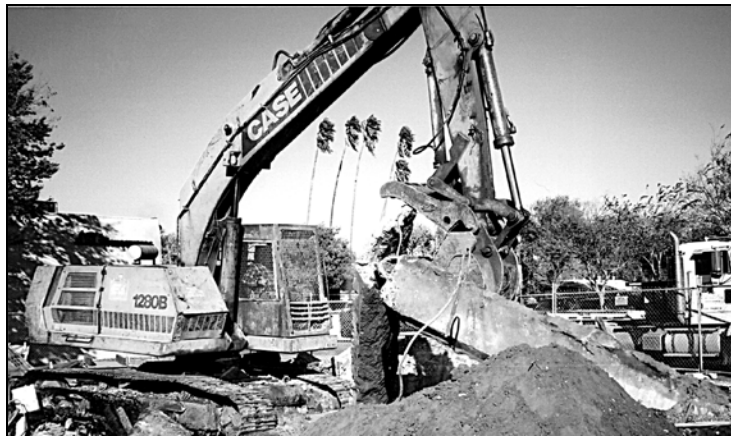
13.24. Pulling up a large chunk of foundation.
