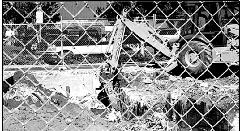
13.23. Jackhammer machine breaking up a basement wall.
