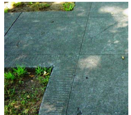
Edge Markings, 600 Block
