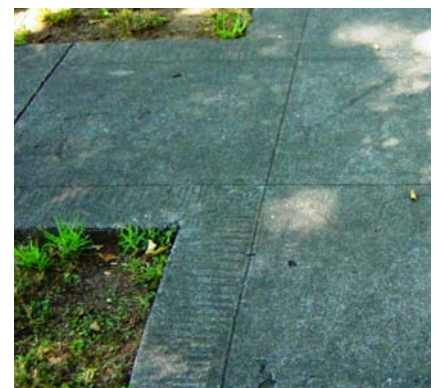
Edge Markings, 600 Block
