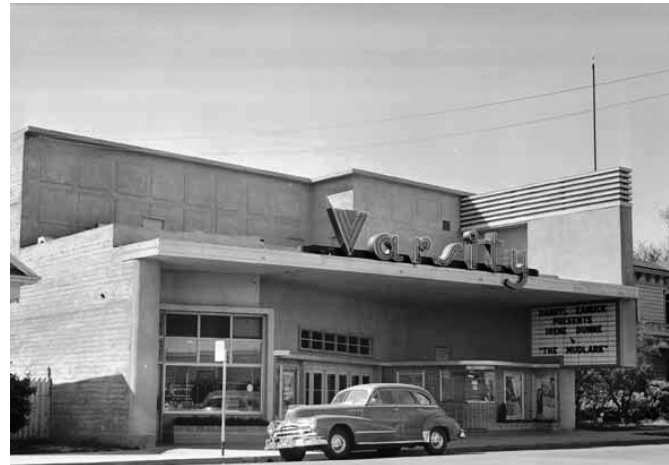
The Varsity as it appeared “new” in 1951. Of special note are the marquee sign out over the sidewalk and the windows above the doors. (Photo from John Lofland, “Davis 1910s—1940s,” original in UCD Special Collections, Eastman’s Originals Collection.)
