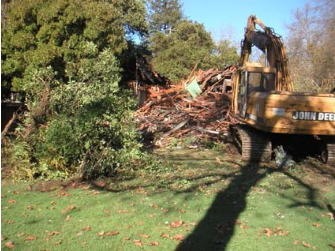
Photograph of the Demolished 319 Russell Blvd.
