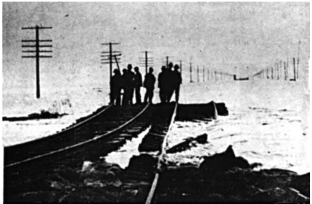
THE FLOOD NEAR DAVISVILLE, circa 1900. This photograph shows the raging current that washed out the railroad tracks east of Davisville during one of the recurring floods which eliminated all but nautical modes of transportation between that place and Sacramento. Silhouetted against the flood waters are a group of local gentlemen who fearlessly ventured beyond the bulwark of sandbags, lower right. Although this pictorial record does not exactly portray the advantages of living in
